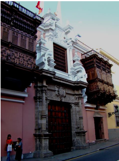
Figure 2: Outside the Celosias, Torre Tagle Palace in Lima, Peru
