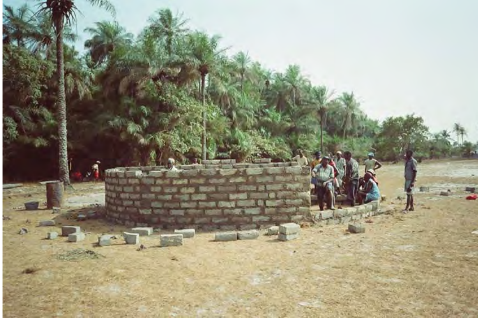
Figure 2. Construction on the first guesthouse gets underway. 2007. Photograph by author.
