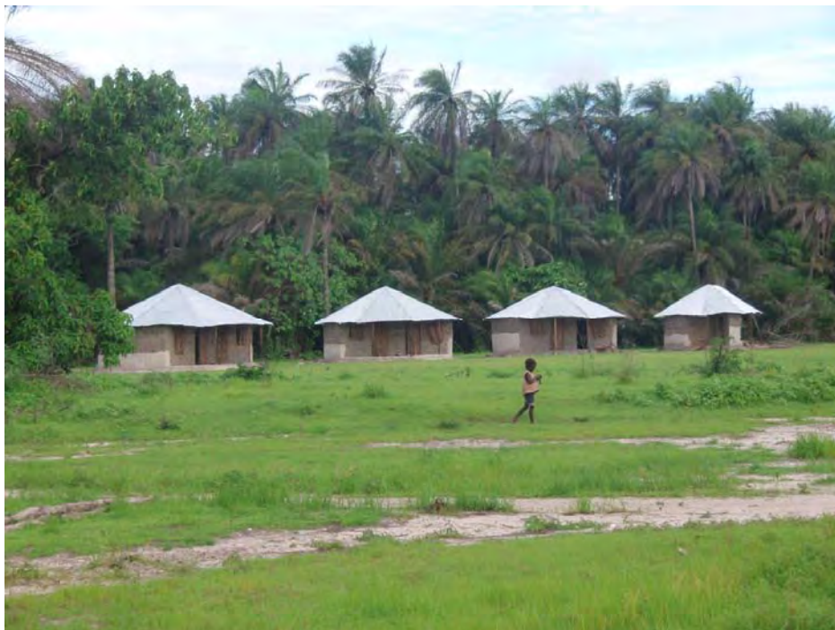
Figure 3. Construction is just about complete. 2010. Photograph by author.
