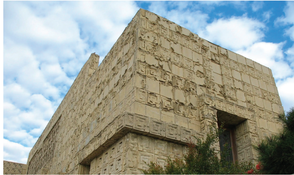
Figure 16. Ennis House . "Ennis House." SGH, September 20, 2021. https://www.sgh.com/project/ennis-house/ .
