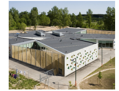
Figure 2.44 - Kindergarten Lotte https://archello.com/project/kindergarten-lotte
