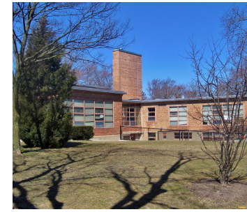
Figure 2.42 - Crow Island School https://www.claasshaus.com/blog/10-things-crow-island-elementary-school
