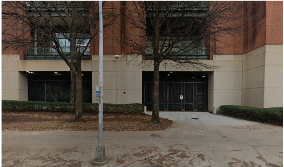
Figure 7.7: Original west side gates, new entrances combine the two to create a wider entry/exit point for the first floor 14
