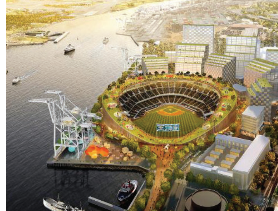
Figure 2.3: Shows aerial image of Oakland Stadium by BIG, shows integrated park space 6
