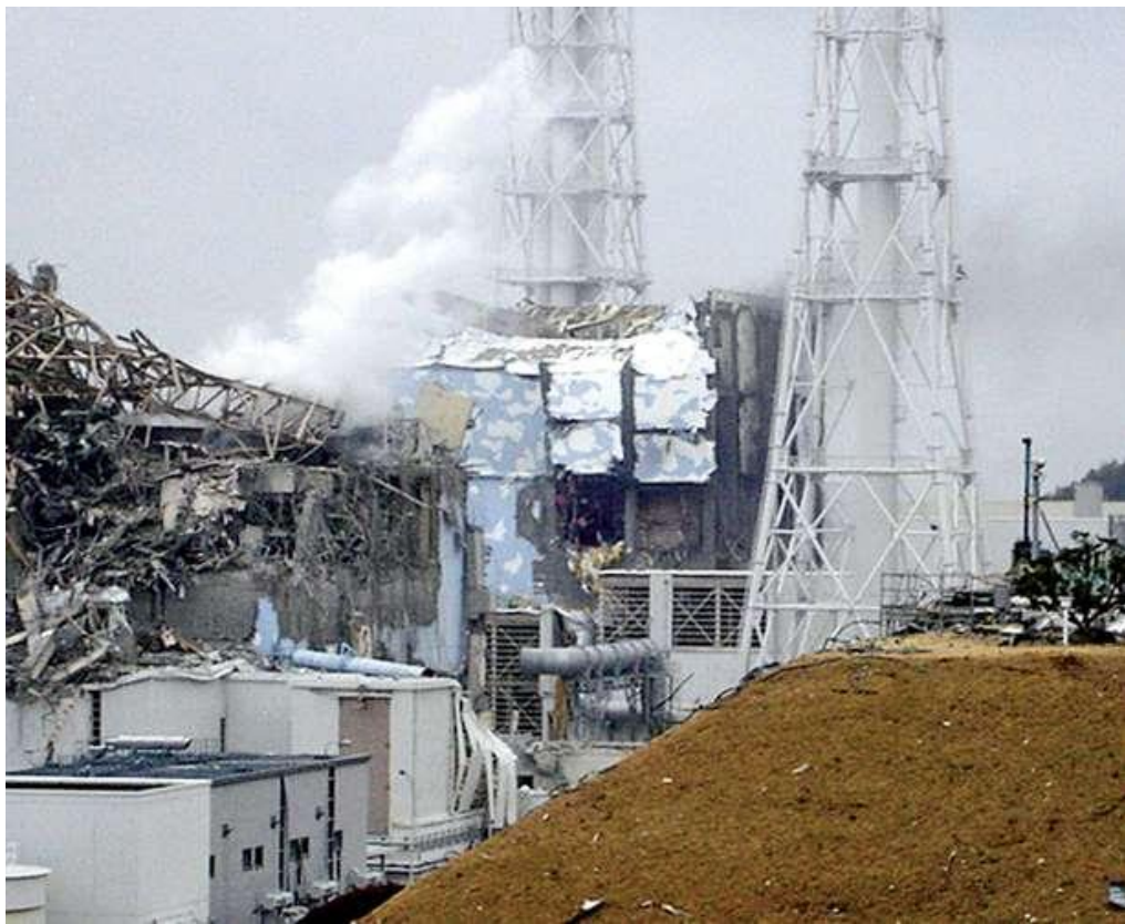
Figure 1.1 Damage at Fukushima Daiichi Nuclear Power Plant, run by Tokyo Electric Power Co.—Kyodo News/AP
