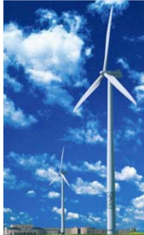
Figure 1: NEG Micon Turbine in Moorhead Minnesota (DOE)
